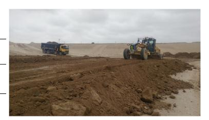
Geo-Logic Peru (GLP) provided assurance and quality control of the construction of dams in tailings facilities 1-5 for Compañia Minera Miski Mayo S.R.L. The project includes the construction of dams around the facility initially built by the client, as well as the installation of the projected geotechnical instrumentation.
