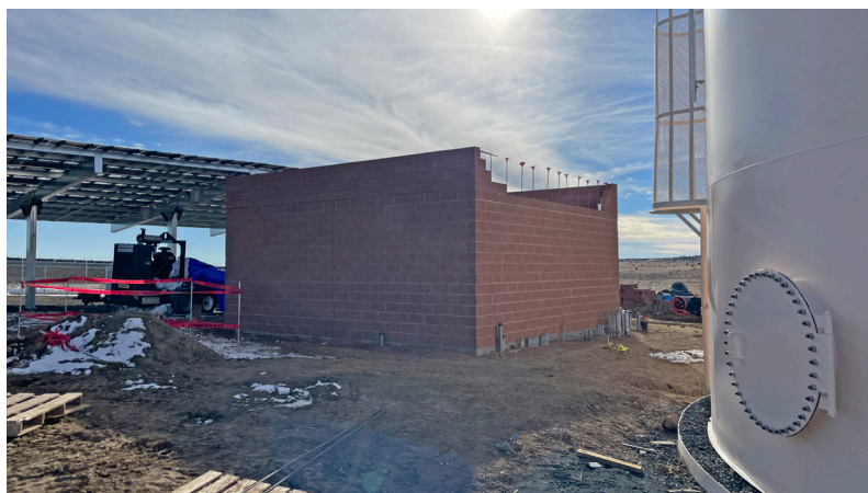
Construction of the regional water system for the Hopi Utilities Corporation
