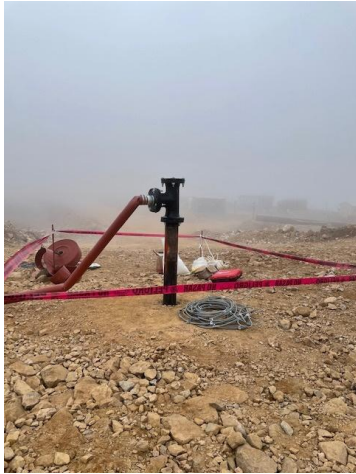
Figure 6. Typical low pressure injection well head
