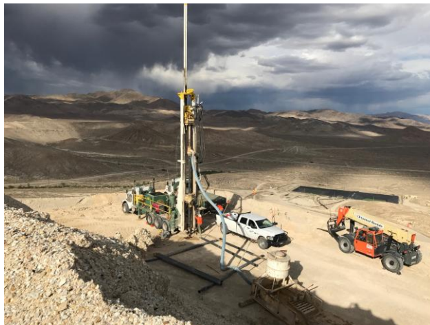
Figure 3. Typical dual rotary drill rig
